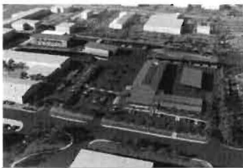
Greenwood Village Public Works Facility Expansion
