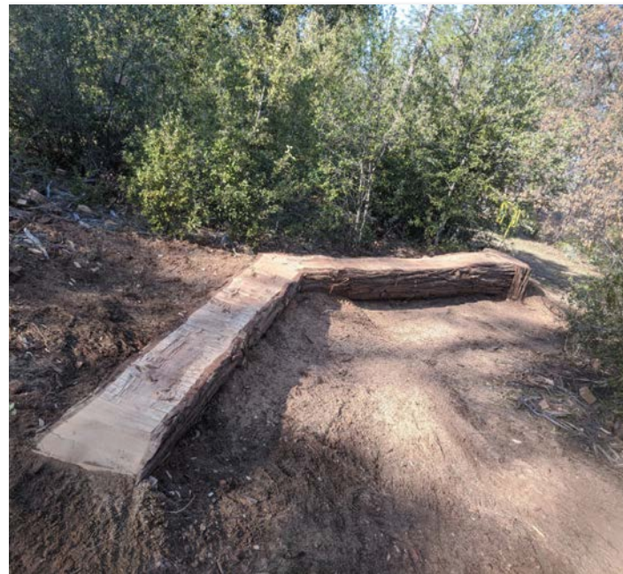
SKINNIES AND LOG RIDES: These elevated and narrow riding surfaces help to develop balance skills. These elements can be built from fallen trees, split logs, milled planks, or dimensional lumber. They can also be straight, curved, or angled.
