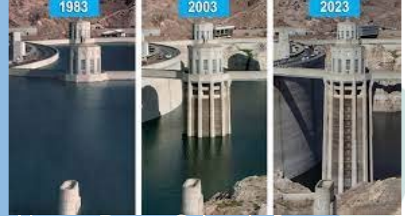
Hoover Dam – Colorado River
