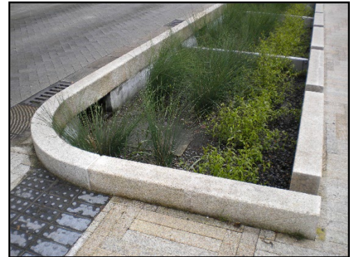
Fig. 3-27-BB: LID stormwater management feature
