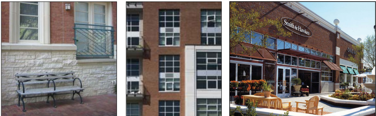
Fig. 3-27-W: Mix of building materials
