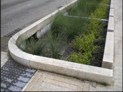
Fig. 3-27-BB: LID stormwater management feature
