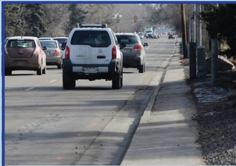
4-foot sidewalk attached to roadway Acera de 4 pies conectada a la carretera
