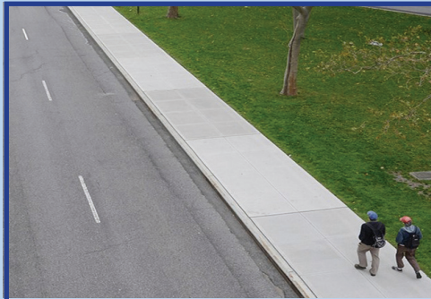
12-foot shared use path attached to roadway for use by pedestrians and bicyclists Camino de uso compartido de 12 pies adjunto a la carretera para uso de peatones y ciclistas
