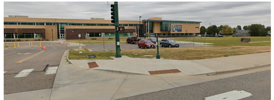
FIGURE 4. SOUTHGATE INTERSECTION - COMPLETE AND ADA COMPLIANT CURB RAMPS.
