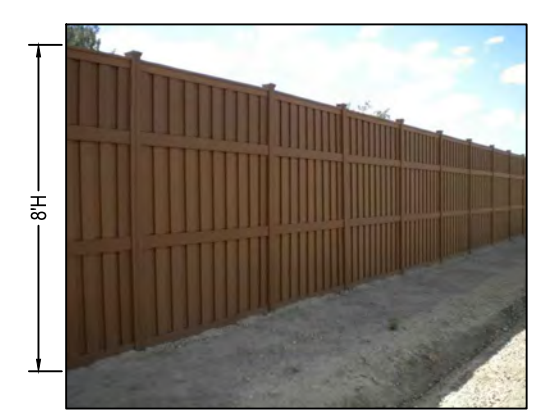
PRIVACY FENCE DETAIL (TREX SADDLE COLORED 6" FENCE, OR SIMILAR) *1300' PROP. FENCE DIST.
