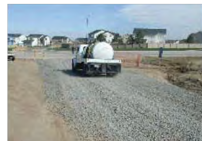
Photograph DC-1. Water truck used for dust suppression. Photo courtesy of Douglas County.
