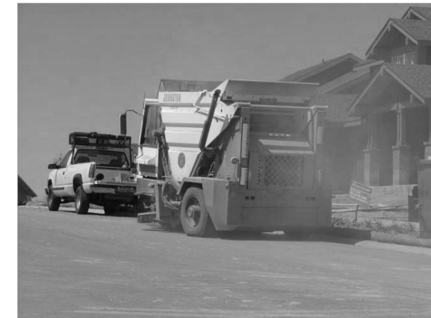
Photograph SS-4. A street sweeper removes sediment and potential pollutants along the curb line at a construction site. Photo courtesy of Tom Gore.
