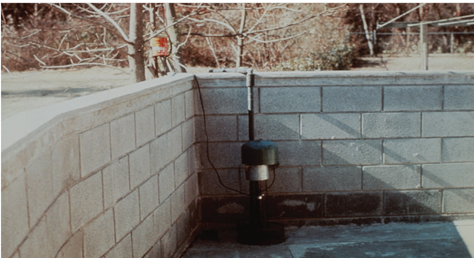
Figure 8-6. Small patio floodwall with sump pump.
