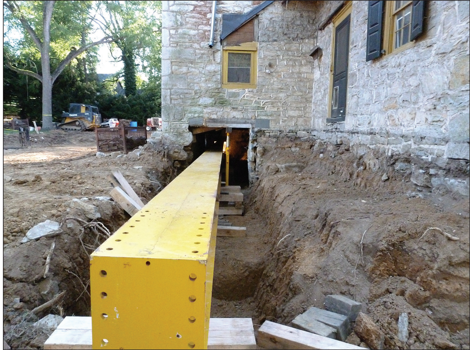
Figure 6-3. Pathways for lifting beams (photo courtesy of Wolfe House Movers).
