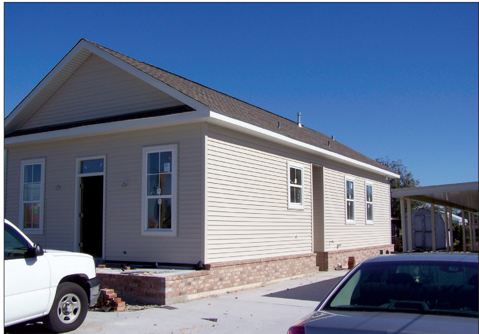
Figure 6-9. Typical mitigation reconstruction project.
