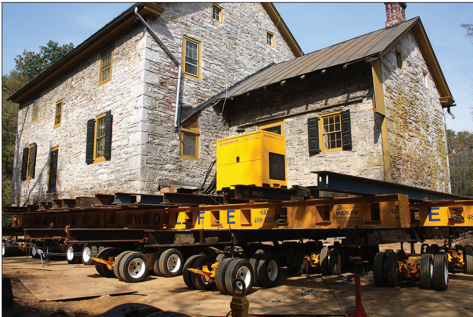
Figure 6-6. Trailer wheel sets are placed beneath the lifting beams (photo courtesy of Wolfe House Movers).
