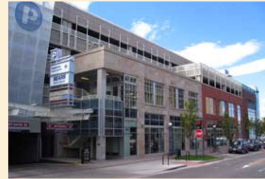
Parking wrapped with street level retail
