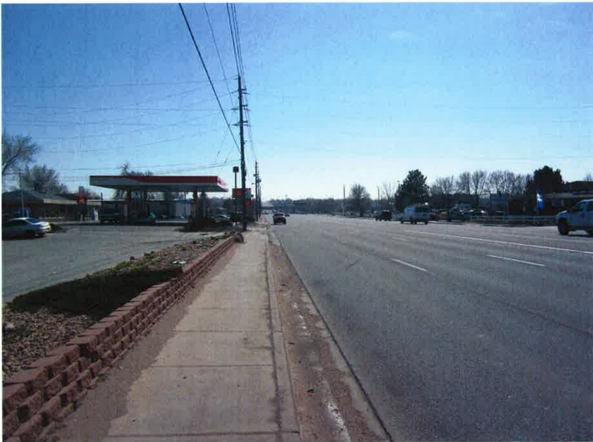
Figure 20: Typical sidewalk section on Federal Boulevard looking south near West 64 th Avenue
