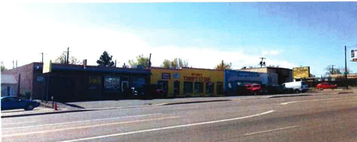
Figure 4: Typical commercial building strip development pattern located near W. 65 th Avenue
