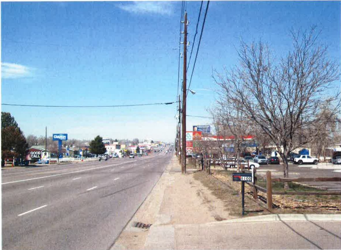
Figure 21: The corridor lacks overall sidewalk connectivity, as depicted here looking north near West 61 st Avenue
