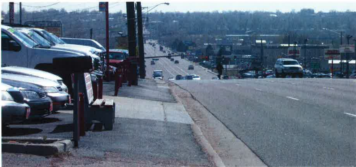
Figure 24: Frequency of driveway curbs cuts impacts usability of pedestrian facilities near 65 th Avenue
