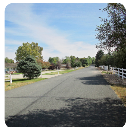
Local Road in District
