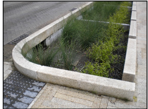
Fig. 3-27-BB: LID stormwater management feature
