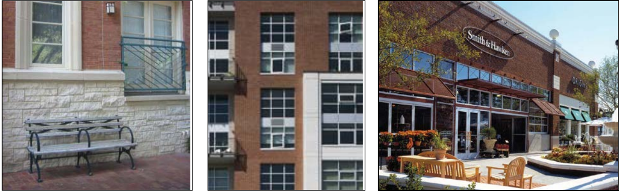
Fig. 3-27-W: Mix of building materials
