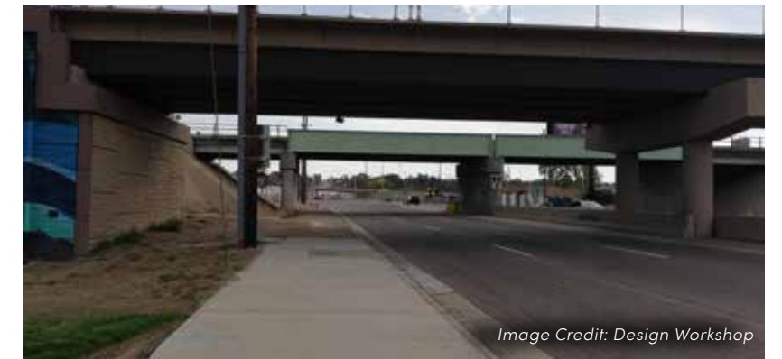
Figure 45: Federal and West 60th Avenue Looking South
