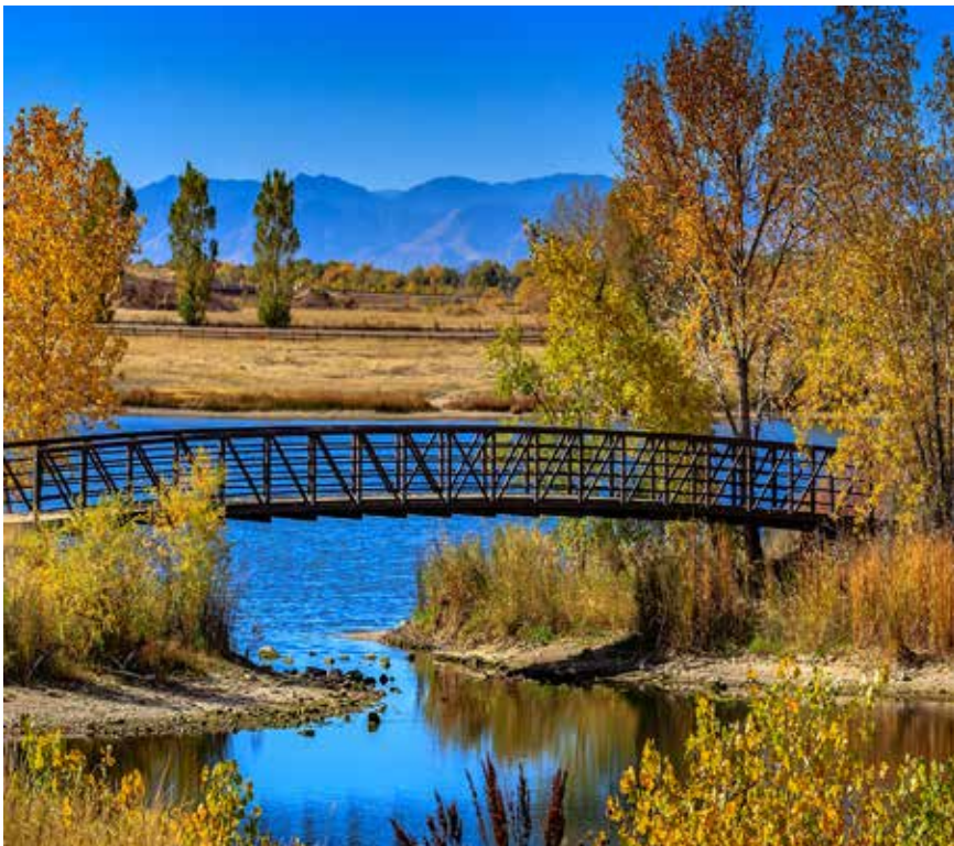
Riverdale Regional Park Bridge
