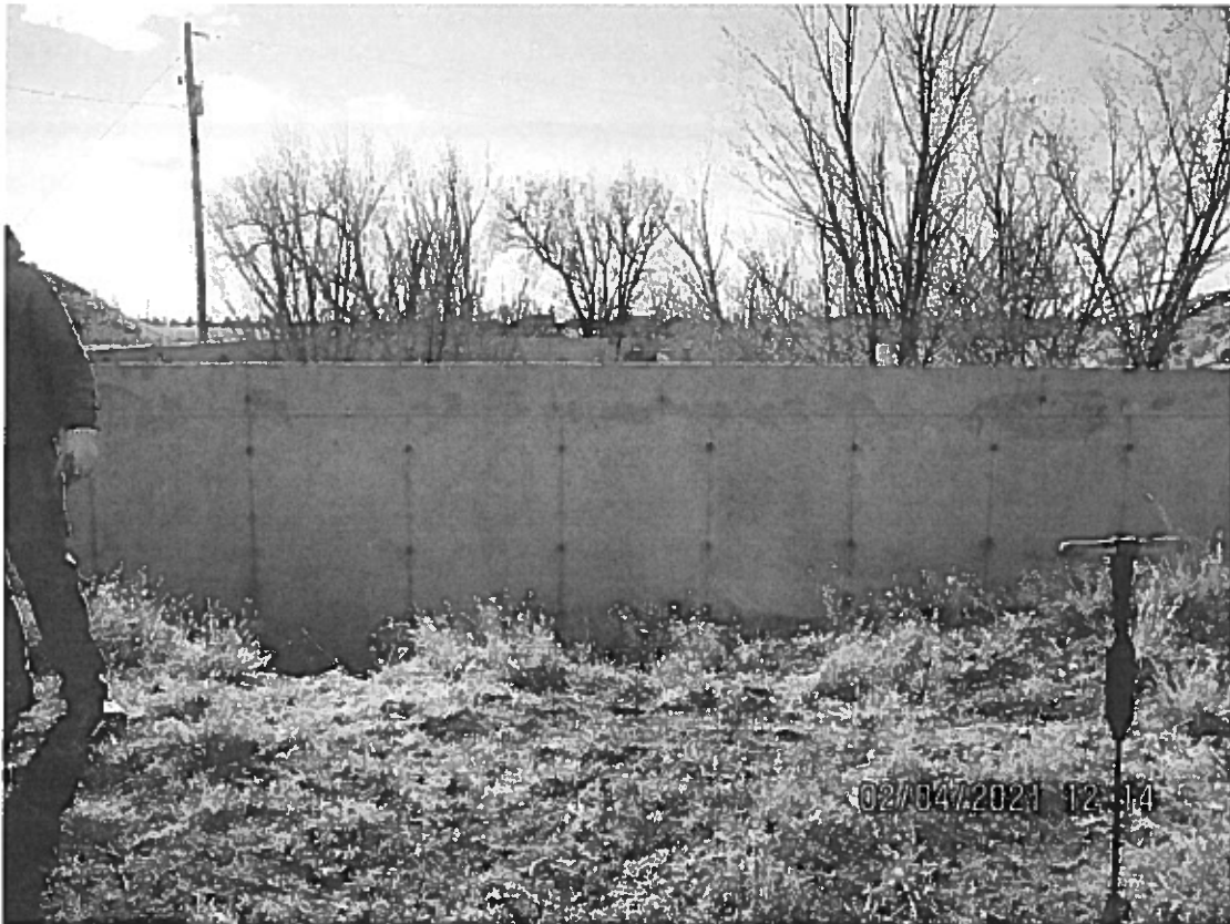
Foundation present at 2580 Xmore Mile Road, Byers, CO 80103
