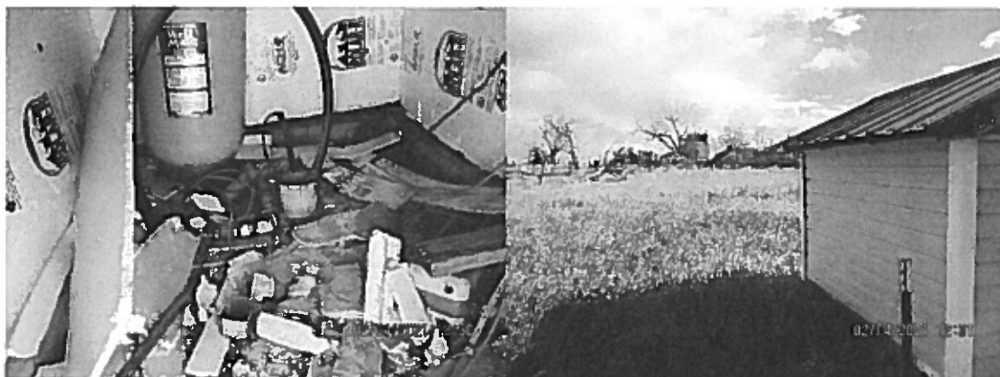
Non-Functional Well Shed located 160' west of the foundation
