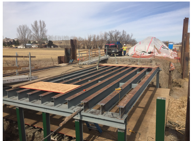
Structural steel repairs, March 2018
