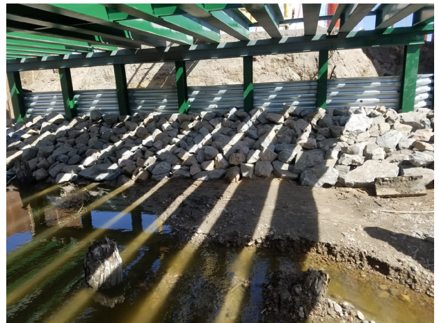
Completed work under the deck, April 2018
