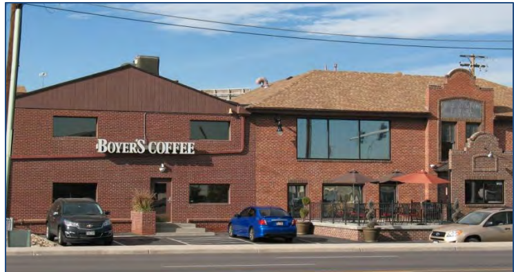
Boyer's Coffee at 73 rd Ave. and Washington St. is an existing example in Welby that has a "beehive concept" model with both retail and distribution in one location.
