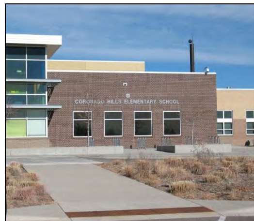
Coronado Hills Elementary School north of Coronado Parkway at E. 83rd Place.
